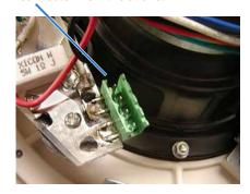
Connect the plug from the can (or from the conduit wiring, see Figure 5) to this socket on the loudspeaker assembly.
